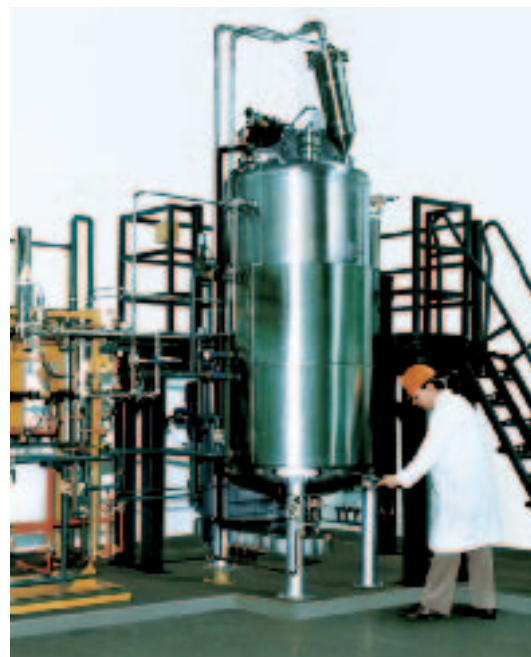
FIGURE 14-14 Industrial-scale fermentation. Microorganisms are cultured in a sterilizable vessel containing thousands of liters of growth medium—an inexpensive source of both carbon and energy—under carefully controlled conditions, including low oxygen concentration and constant temperature. After centrifugal separation of the cells from the growth medium, the valuable products of the fermentation are recovered from the cells or from the supernatant fluid.
